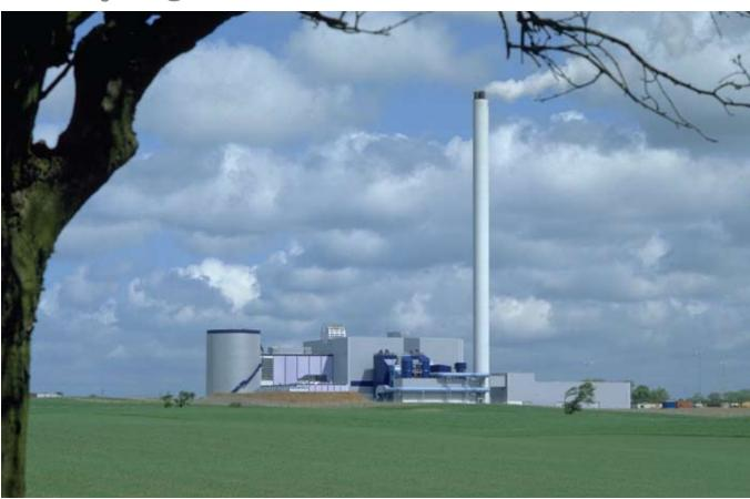
Måbjergværket is the first CHP plant in Denmark to use a fuel combination consisting of waste, wood chips, straw and natural gas.
