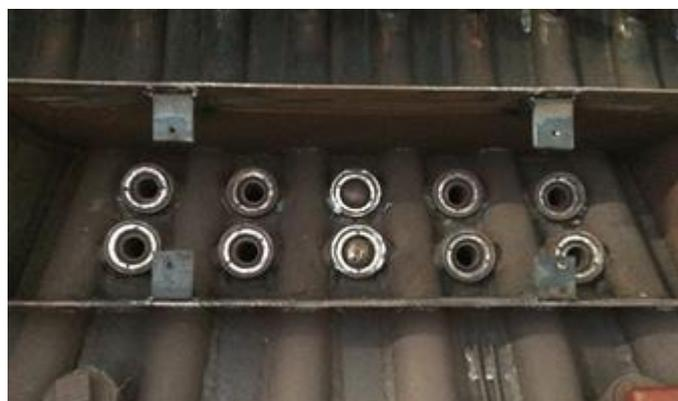
Figure 2. Secondary air nozzles on back wall (2<sup>nd</sup> level)
